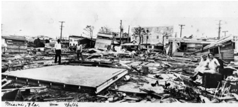
Damage from the Great Hurricane of 1926
